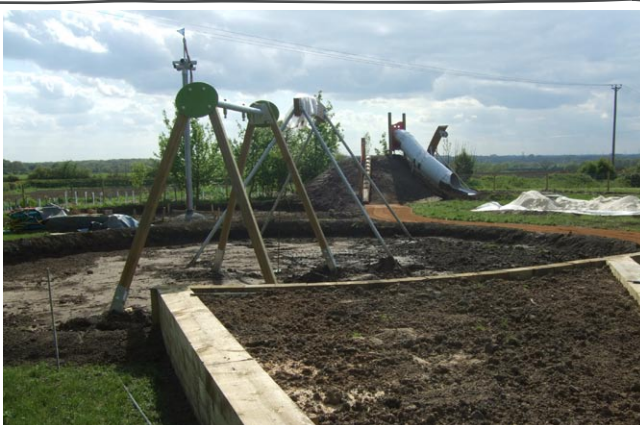
Construction at one of our sites
